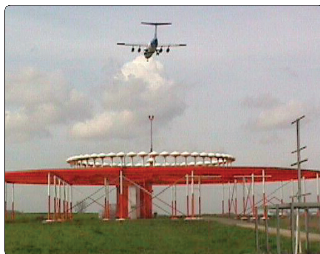
Figure 11-119. A VOR with DME ground station.
